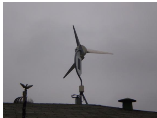
Overall view of turbine
