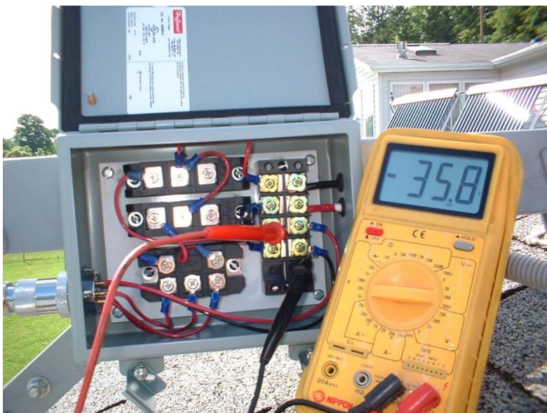
Image 2 – Testing the connections
